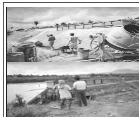
The Labo River Control structure undergoing repair and maintenance.
