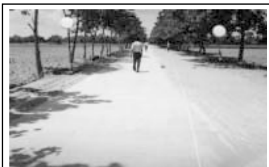
The Cagayan-Apayao concrete road at Mungo section is a big boost to the province's economy.
